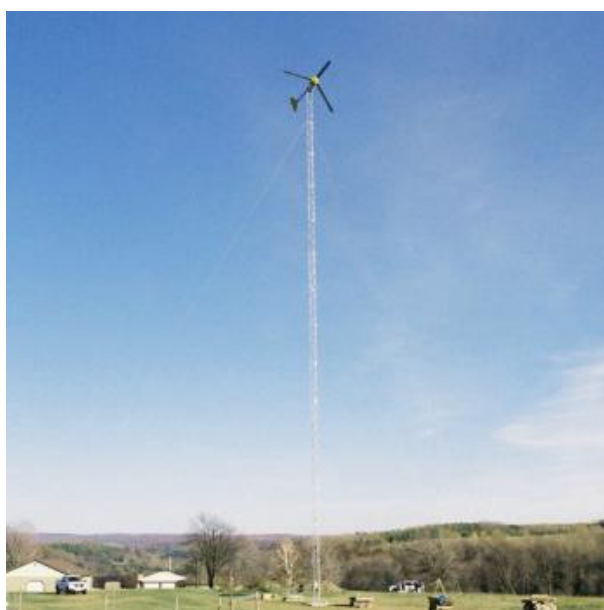
Figure 6. A 10 kW turbine on 140-foot freestanding lattice tower for residential and/or agriculture use [131]
